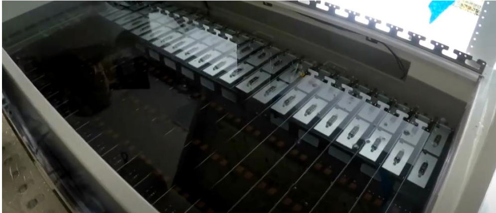
Figure 6 - Several Servers Immersed in Liquid
