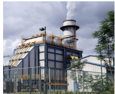
Energy companies are building physically accurate industrial digital twins to reduce unplanned downtimes through predictive maintenance.
